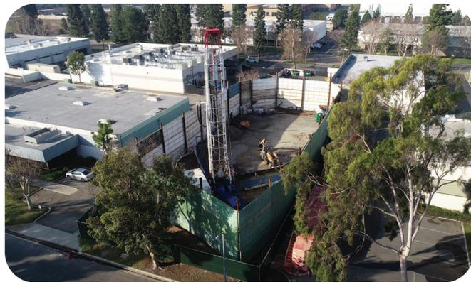
Construction is currently under way for two new potable (drinking) water wells. The 1,000-foot deep wells will allow Mesa Water to increase its local water production capacity, and are expected to be completed in Winter 2022. The two wells will be connected to the existing distribution system by a 4,500 linear foot pipeline.
