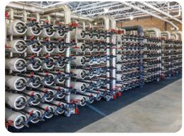
pulled water moves through a sand separator which removes sand and grains. The water then flows through a cartridge filter that removes particulate matter up to 5 micron, about the width of a human hair! Finally, the water makes its way through the vessels which removes the color by pushing the water through a semi permeable membrane element, only allowing the clean water to pass.
