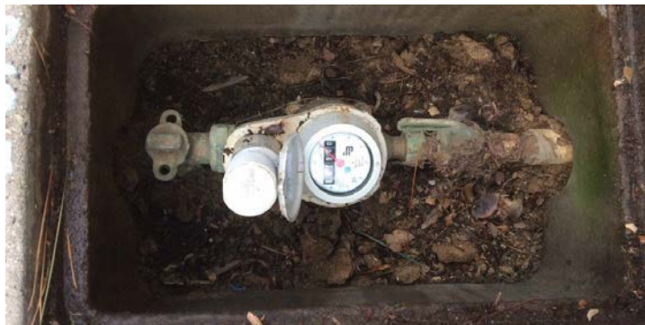
Figure 5 – Small Meter Installation w/CE Device
