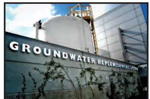
Photo courtesy of Orange County Water District
