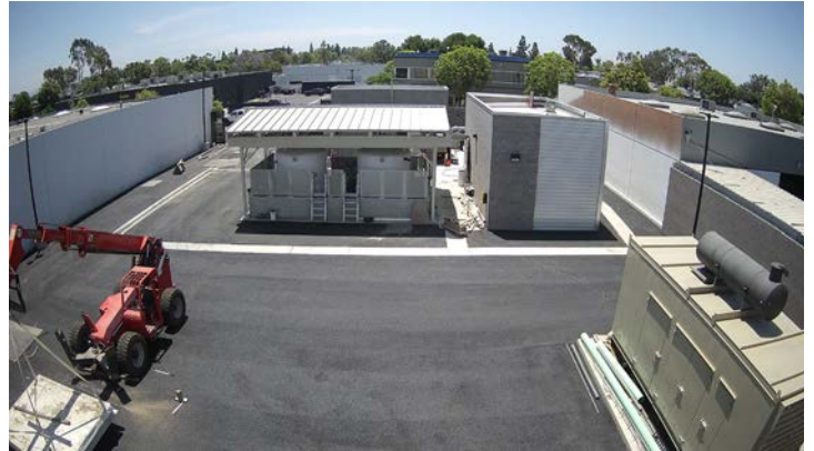
Figure 2. Well No. 12 Site Work
