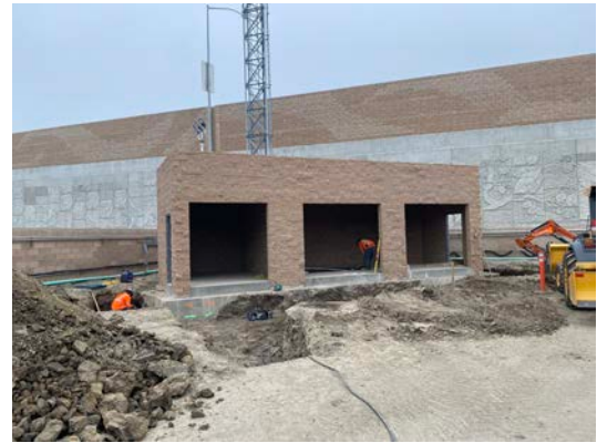
Figure 9. Northwest Storage Building
