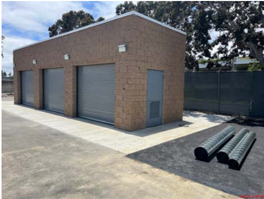
Figure 8. Well Parts Storage Building
