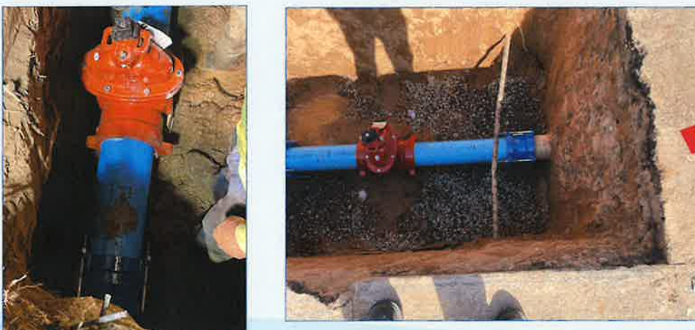
Mainline Valve Replacement Project
