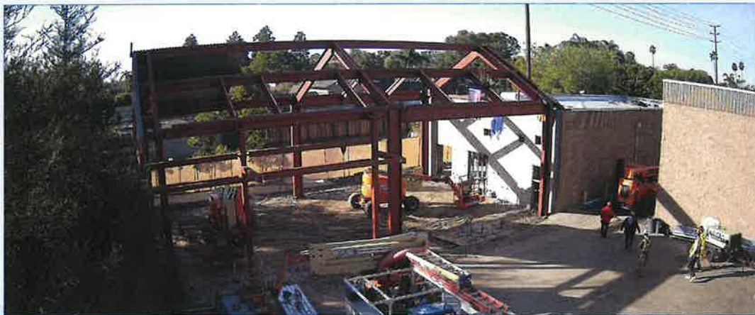
MWRF Administration Building
