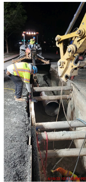
Figure 6. Night work in MacArthur Blvd.
