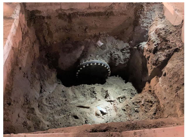
Figure 15. Vault Rehabilitation and Abandonment Project Santa Ana/Del Mar Vault Abandonment
