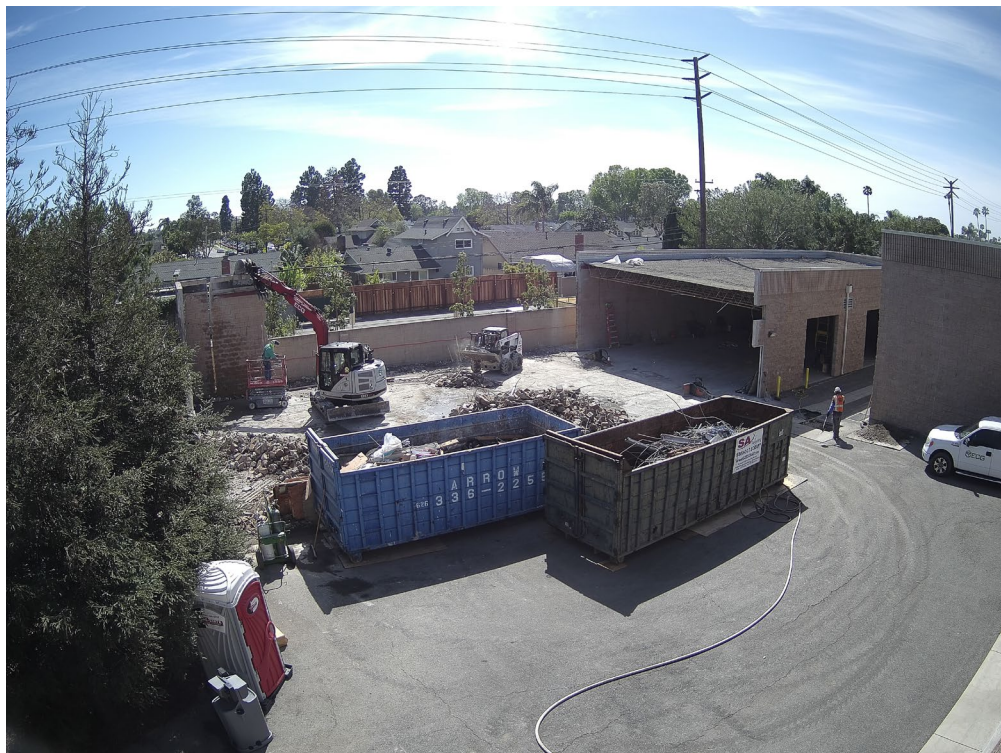
Figure 22. Administration Building Demolition
