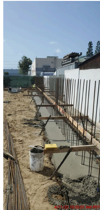
Figure 2. Well No. 14 Perimeter Wall
