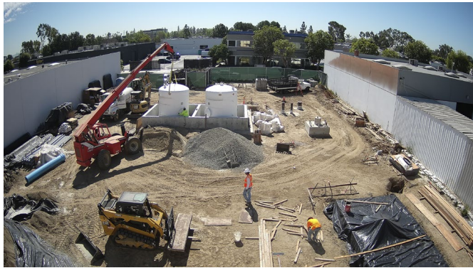
Figure 3. Chemical Tank Installation
