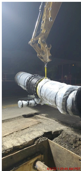
Figure 5. 30-inch Pipeline Installation
