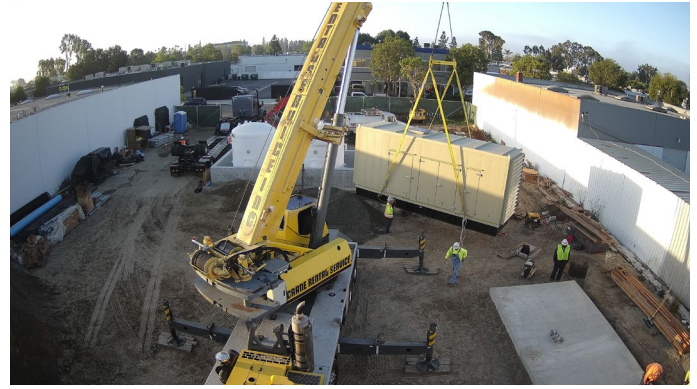
Figure 4. Backup Generator Installation
