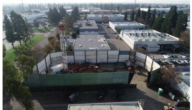
Figure 4. Croddy Well No. 14 Drilling
