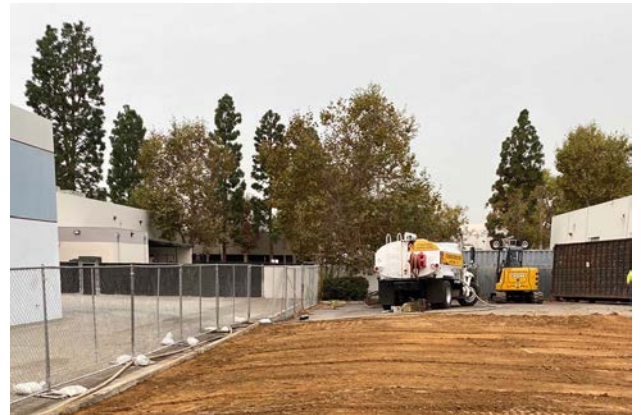
Figure 2. Croddy Well No. 14 Demolition
