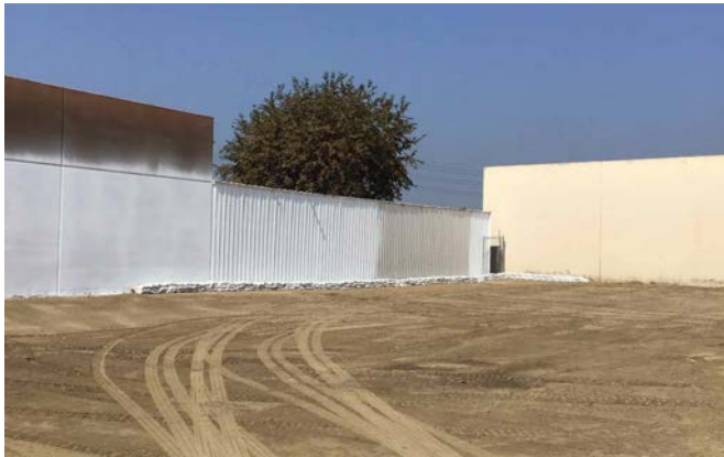
Figure 1. Chandler Well No. 12 Demolition
