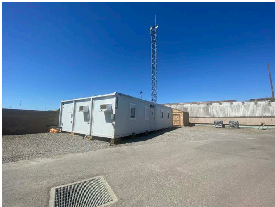
Figure 23. MWRf Temporary Administration Building
