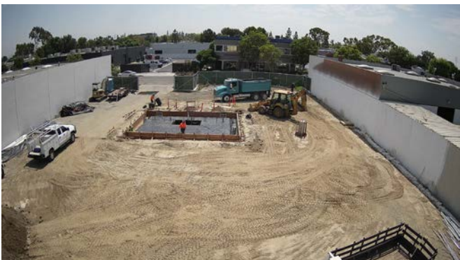
Figure 5. Chandler Well No. 12 Well Equipping
