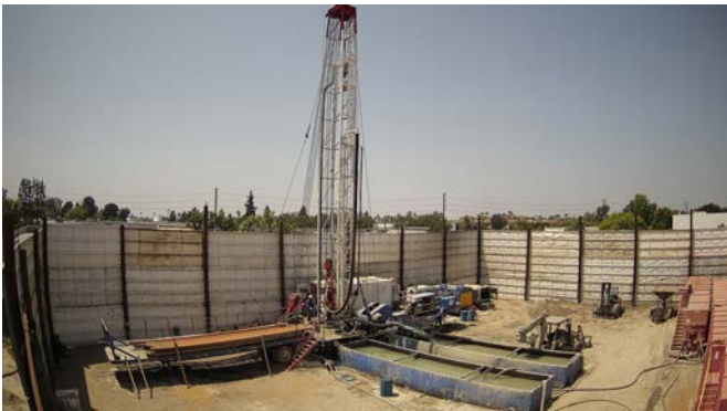
Figure 3. Chandler Well No. 12 Drilling
