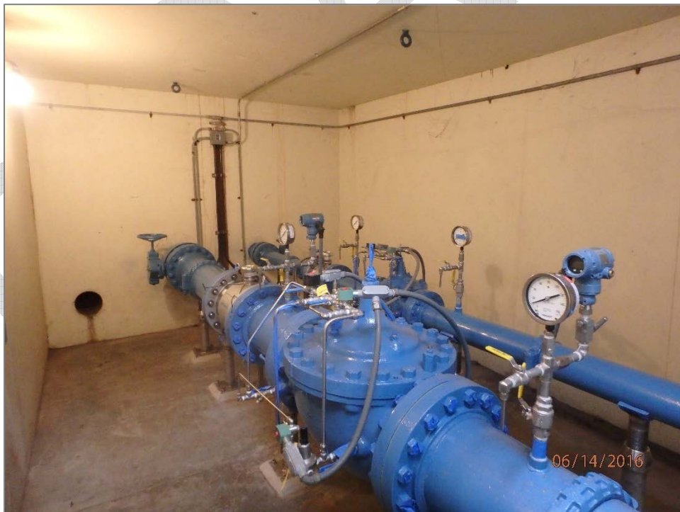
Figure 4-8. Photograph of OC-44, Sub-Turnout 5
