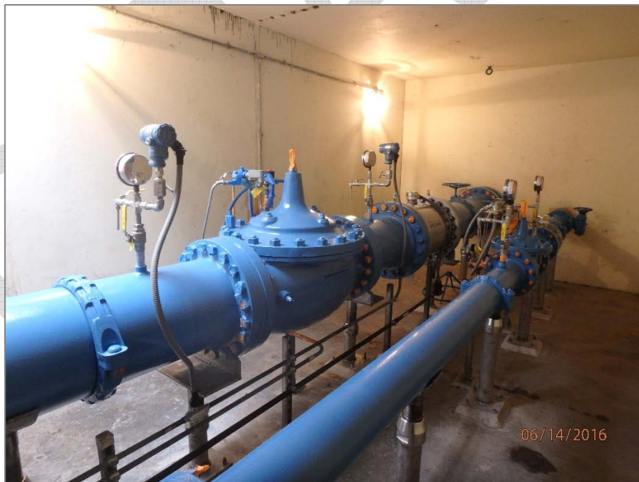
Figure 4-6. Photograph of OC-44, Sub-Turnout 4
